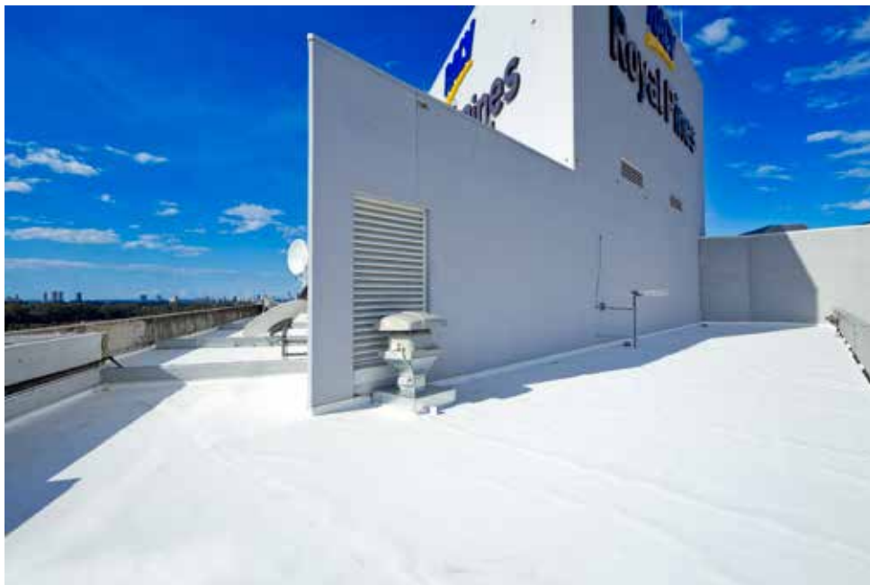
The roof of the RACV Building Royal Pines Resort, Queensland.
