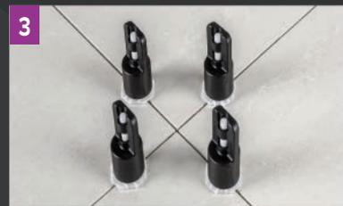
SALS is a Simple Accurate Leveling System for superior wall & floor tile installations. The system will ensure a more precise, **fast installation** eliminating lippage, the unwanted uneven joints between tiles, minimising shrinkage issues and virtually **eliminating any tile surface marks and scratches.**
