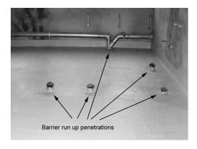
The moisture barrier is applied to all penetrations as well as up the walls to a height of 150mm. All angles and penetrations to be reinforced with ARDEX Deckweb.
